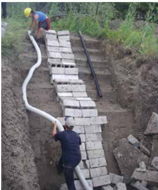
The rock and cinder blocks provide excellent dry hiding places for snakes. This hibernaculum, or home for snakes, was constructed with the help of Stewardship Rangers from Chippewas of the Thames First Nation.
