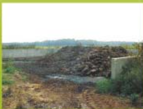
Many improvements to manure storage facilities, such as a roof to be added to this structure, are eligible for funding.
