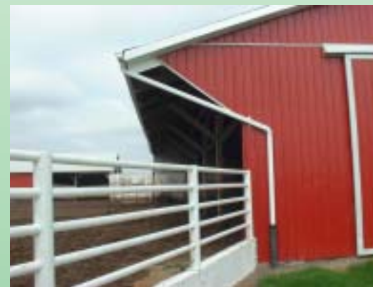
Eaves troughs, diverting roof water away from a feedlot, help to reduce polluted runoff into nearby watercourses.
