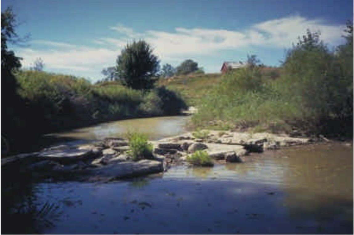
Photo 9. Reach BEAR 10. An abandoned crossing is creating a large backwater area. The channel has begun to circumvent the crossing by eroding away the left bank.
