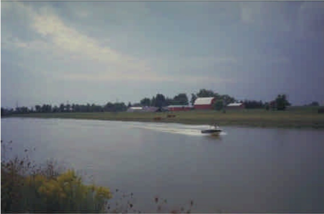
Photo 1. North Sydenham, Reach NS-1. The channel is wide and deep with no apparent morphological structure. The wakes from boat traffic have historically contributed to bank erosion at this location.
